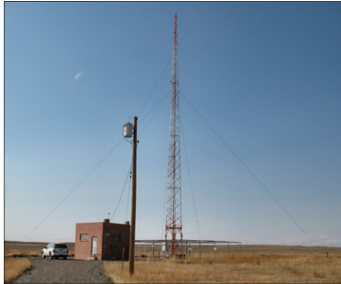
Figure 6-31. Non-Directional Beacon (NDB) facility
