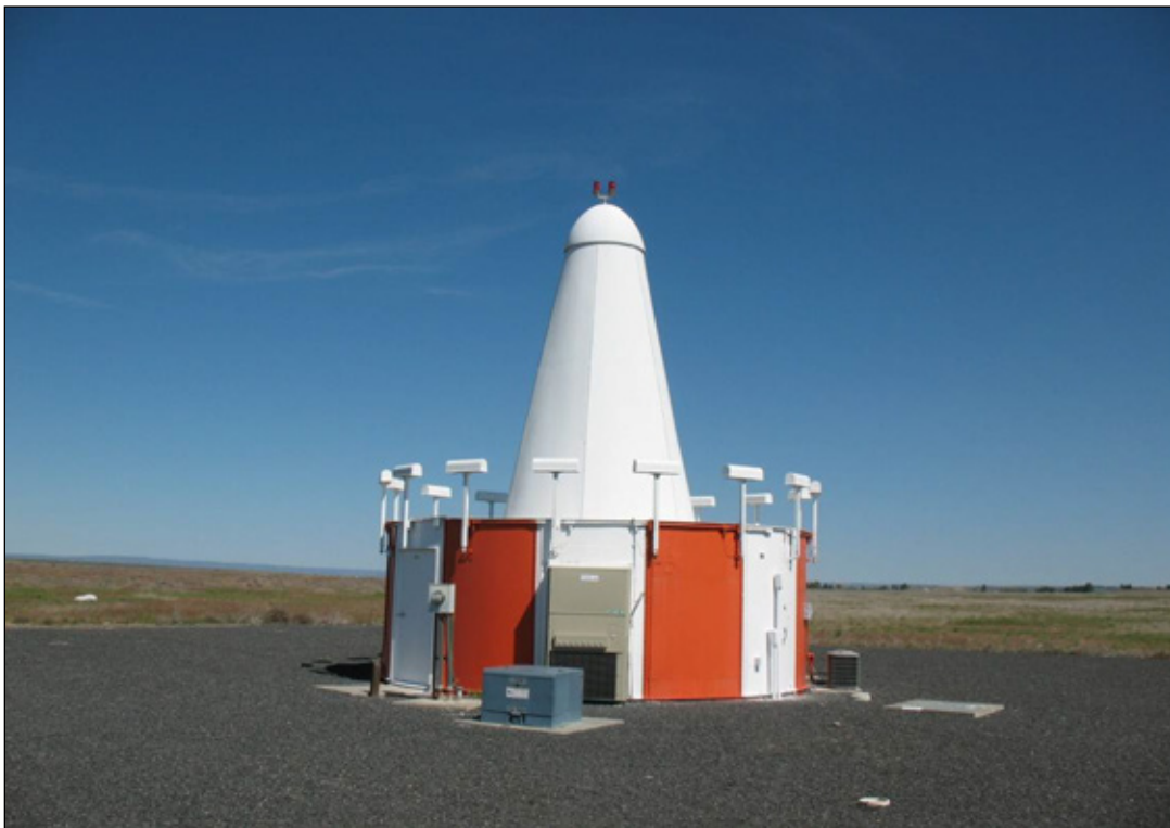
Figure 6-28. Terminal VOR (TVOR) facility
