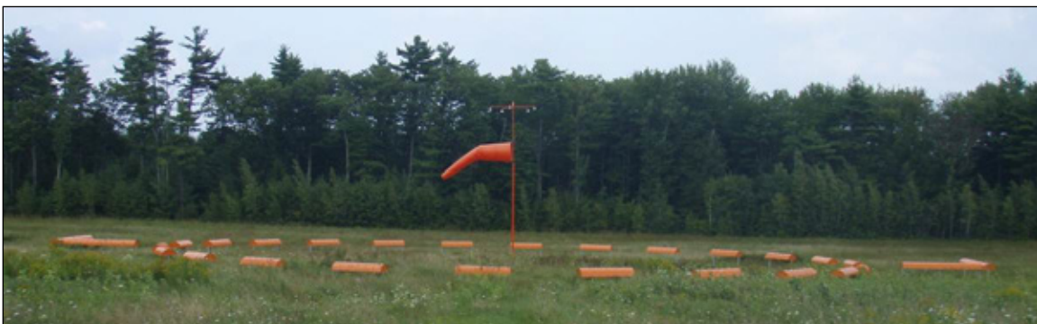
Figure 6-32. Segmented circle and wind cone
