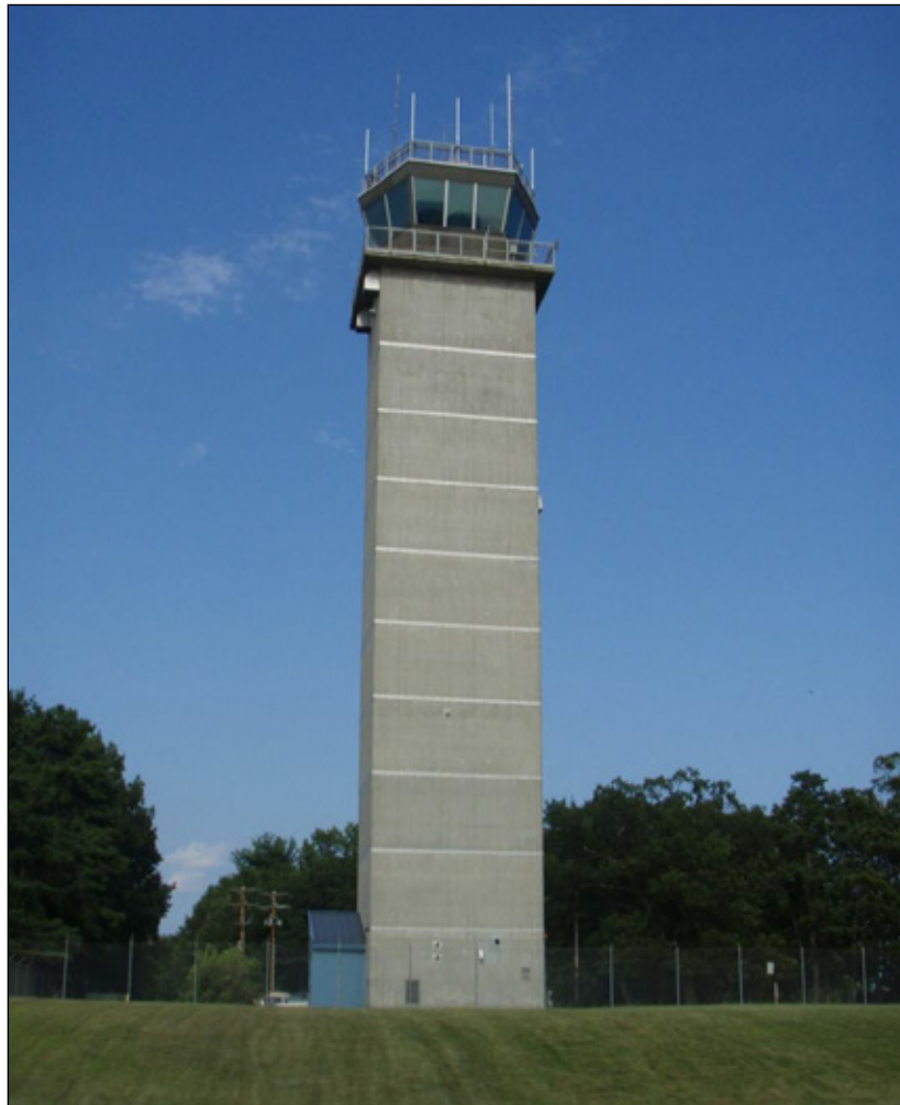
Figure 6-3. Airport Traffic Control Tower (ATCT) facility
