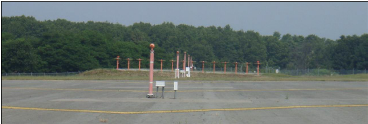
Figure 6-15. Approach LDIN facility
